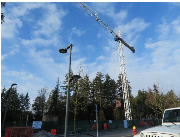
View of the location of the crane at Lot 11.
